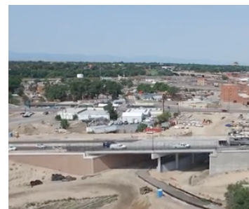
Thomas Phelps Creek Bridge - August 2018
