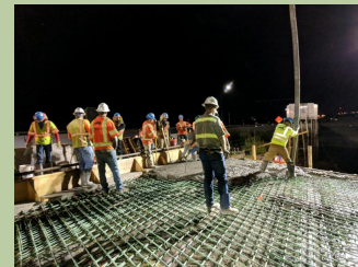
Deck pour at the I-25 bridge over Gruma Drive
