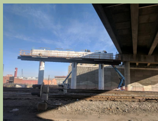
Piers being set at the I-25 bridge over Thomas Phelps Creek
