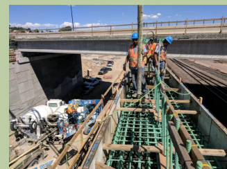
Piers being set at the I-25 bridge over Thomas Phelps Creek
